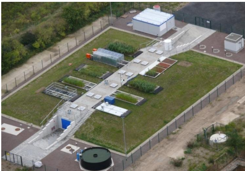
Fig. 2.1-2 The pilot scale plant in Leuna (courtesy of M. Kaestner)
